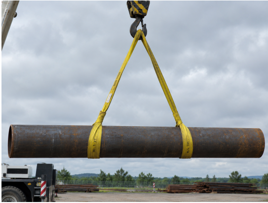
Approved slinging configuration for this load type.
